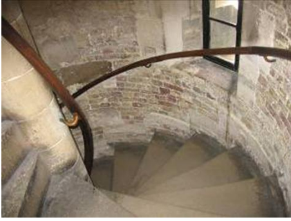
Picture of stairwell at Queen's House, The Tower of London
