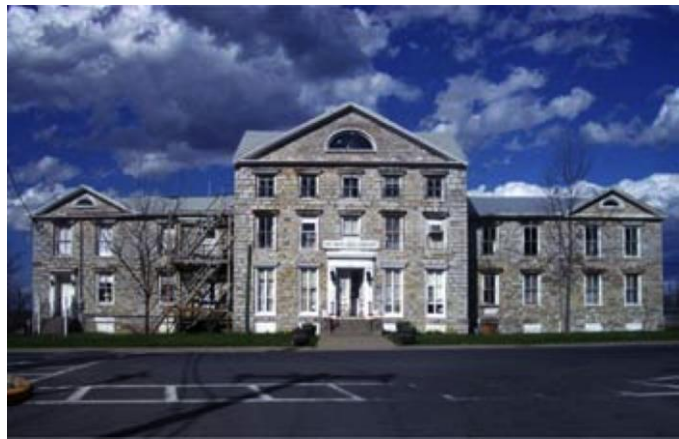
Fig 3. Hudson Area Association Library, New York, reflects the dawn of a new era of window restoration. †
