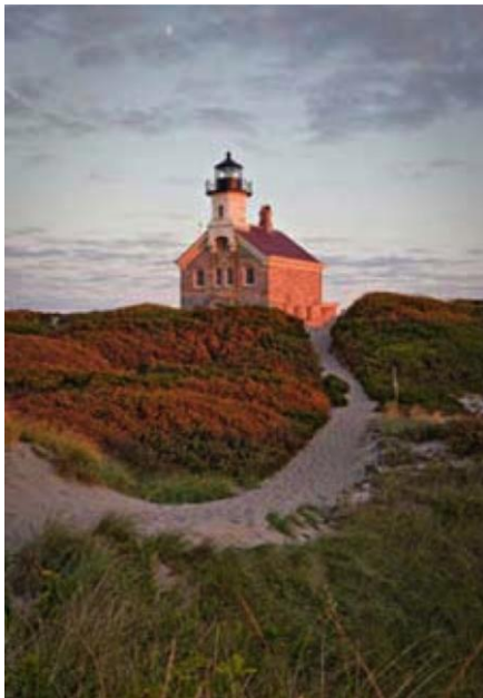
Fig 5. Wind & solar at off-grid Block Island North Light, Rhode Island, provide 100% of the site's energy. †
