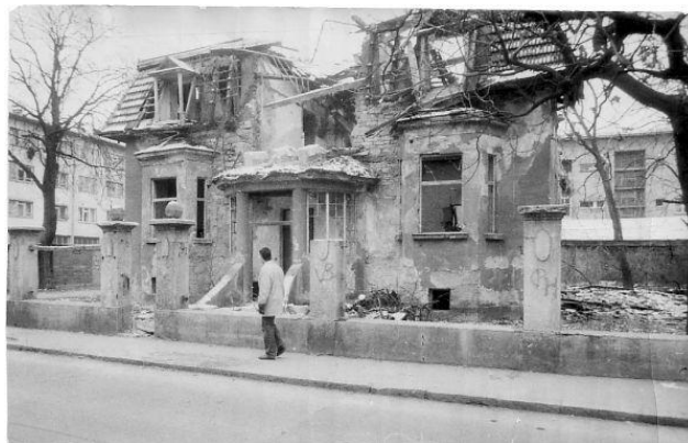
Figure 2: A photograph of Villa Božić in the 1980's, showing traces of time and neglect that gradually led to its demolition (Source: Banjaluca koji ima i koje nema u 1000 slika )
