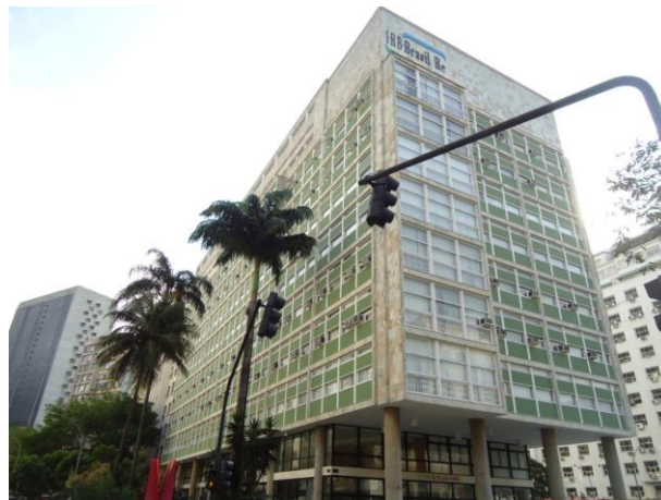
Figure 2. IRB Northeast and Southeast facades
