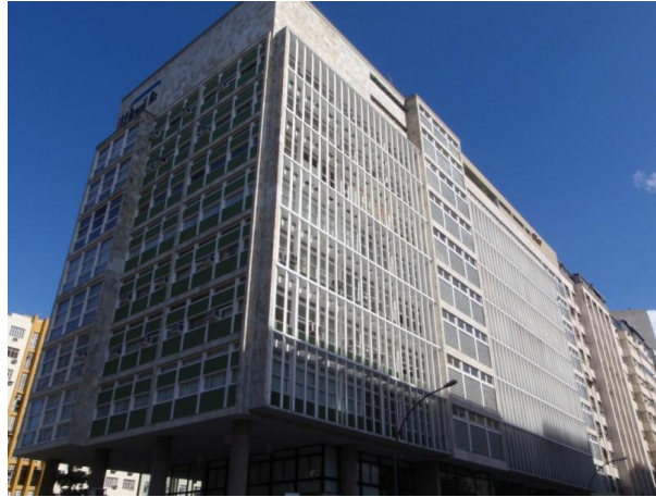
Figure 3. IRB Northwest and Northeast facades
