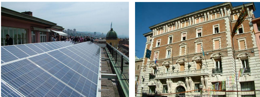
Figure 1: PV system on city of Rijeka Municipality building
