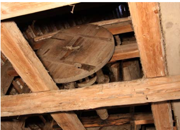
“Alte Schäferei”, historic freight elevator
