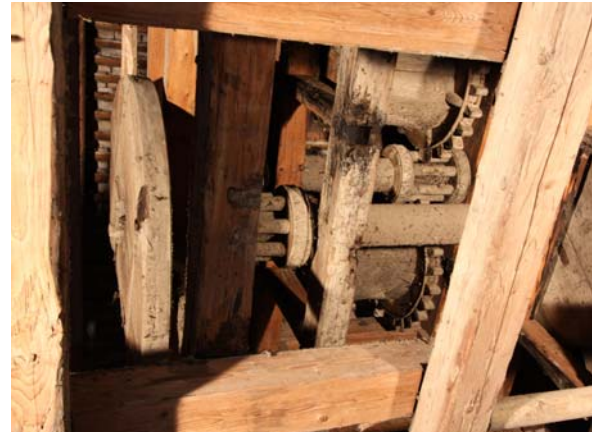
“Alte Schäferei”, historic freight elevator
