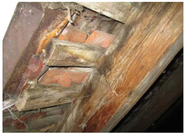
“Alte Schäferei”, Tile and roof framework
