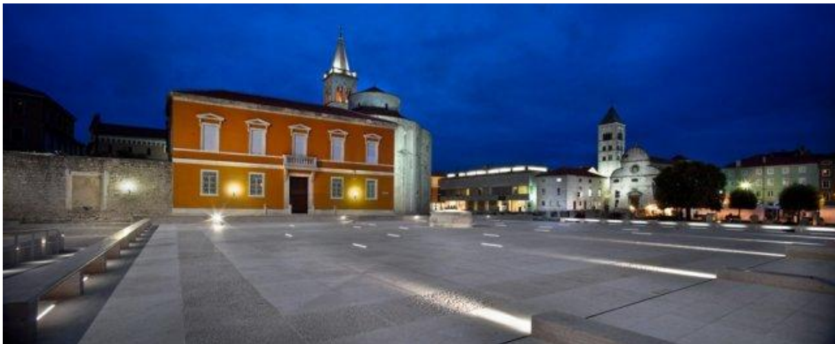
Figure 1. Urban lighting installation on Forum in Zadar, Croatia
