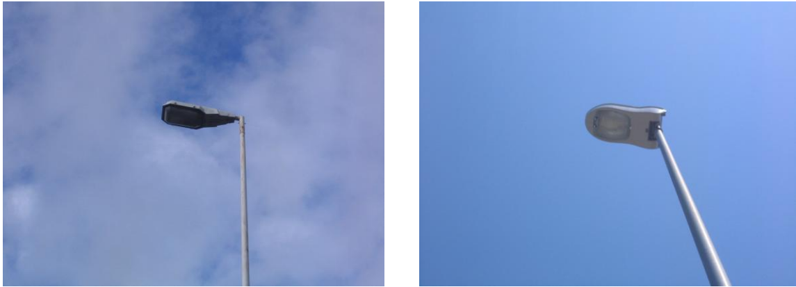
Figure 3. New retro-fitted light fittings with efficient cut-off optics
