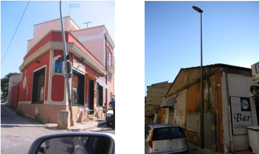
Figure 2. Renewed or new poles
