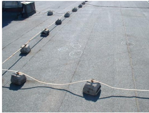
Fig. 3. Photo of flat roof (Jadrolinija Co. building)
