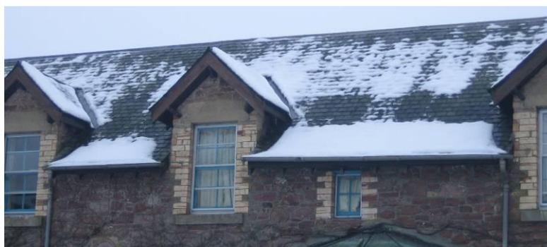
Figure 5. Poor insulation of coombs revealed by snow melt. (Historic Scotland.)
