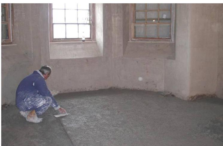
Figure 7 Laying insulating lime hemp floor. (Simpson and Brown Architects.)
