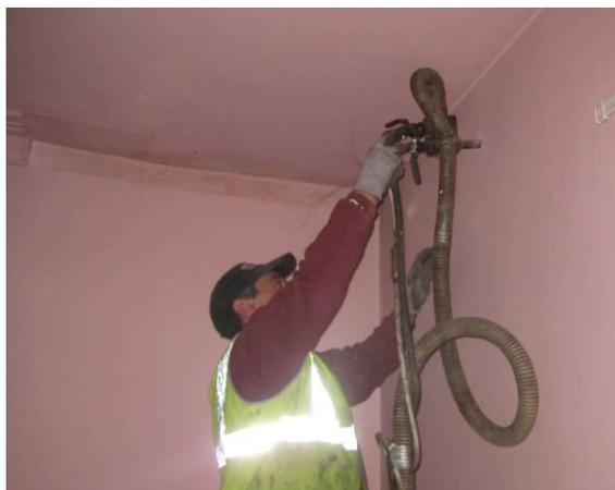
Figure 4. Application of blown cellulose insulation (Historic Scotland).
