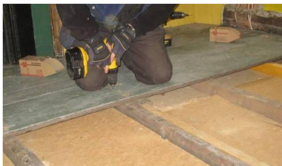
Fig 6. A timber floor being re-laid following addition of insulation board. (Historic Scotland).
