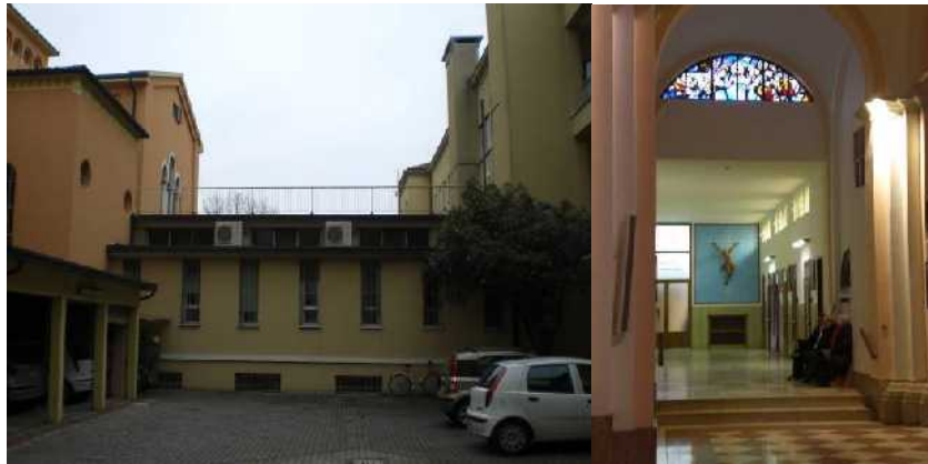
Figure 11. Area subject to demolition and reconstruction
