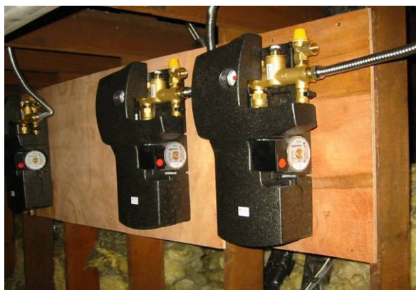
The pump stations (© Lister Housing Co-operative)
