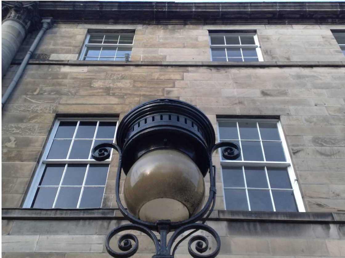
The top-left window of this grade 'A' listed building has slim-profile double-glazing (© Changeworks)
