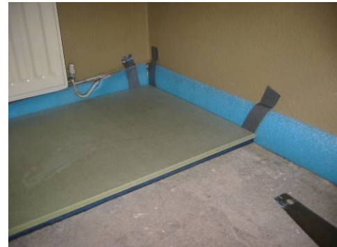
Spacetherm floor insulation being laid (© Changeworks)
