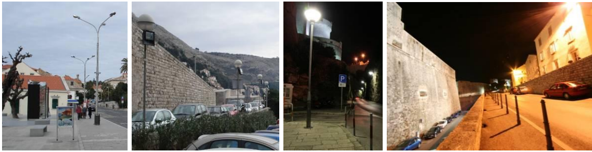
Figure 13. Old lighting situation in surrounding area (around Old City)
